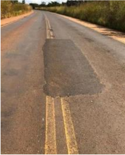
Figura 05 – Remendo
