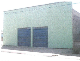
FACHADA DEPOSITO PRINCIPAL
